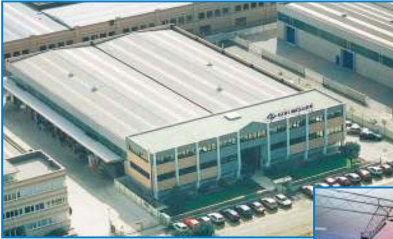
GIVI MISURE's production site in Nova Milanese (Milan), Italy
